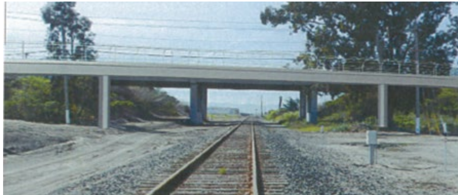
Figure 2. Photo in 2014 Before Construction
