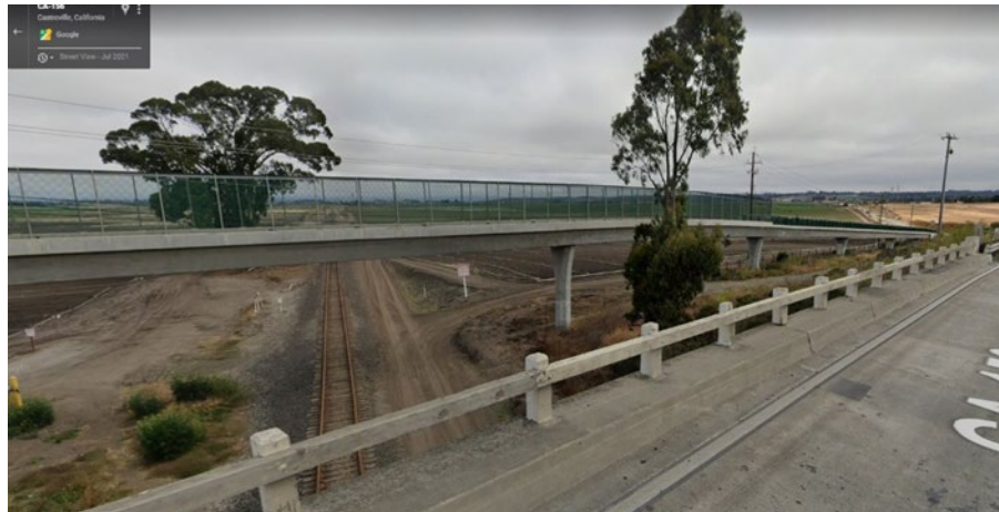
Figure 3. Photo in 2022 After Construction
