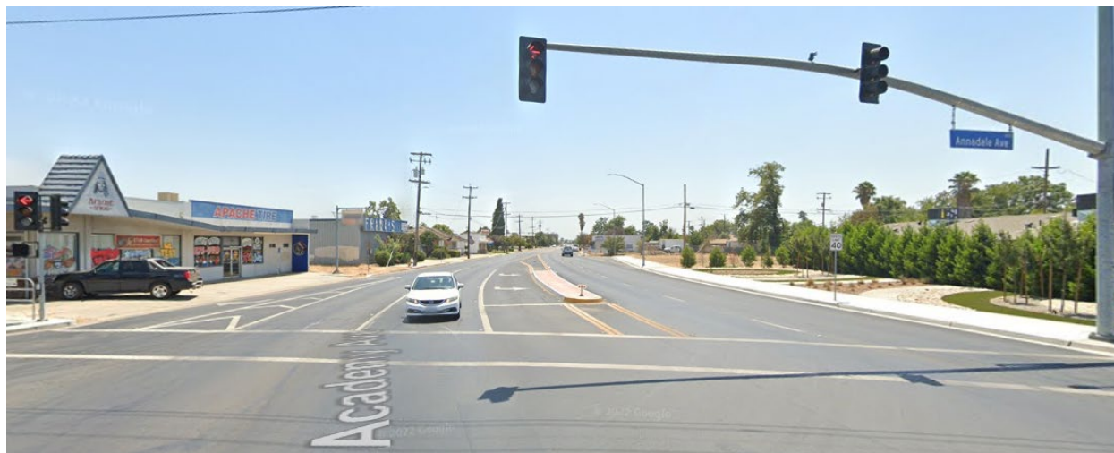
Figure 4. Photo in 2022 After Construction of the STBG Project
