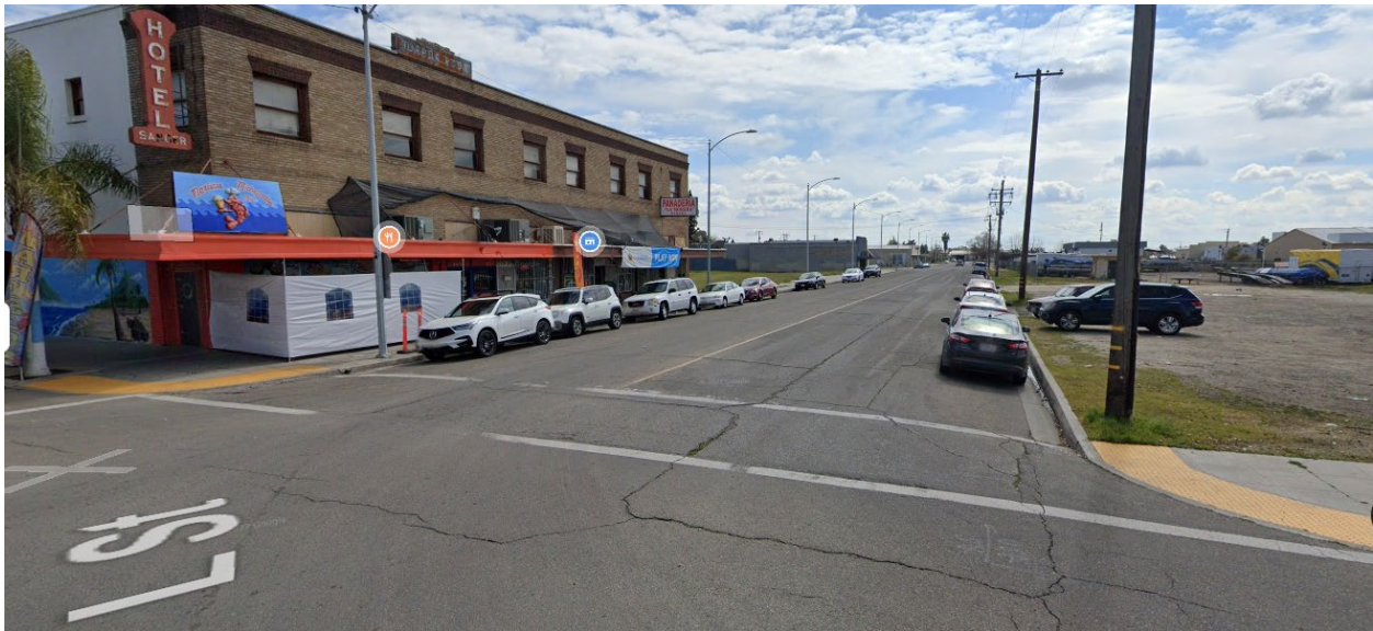
Figure 2. Photo in 2021 After Construction of the ATP Project
