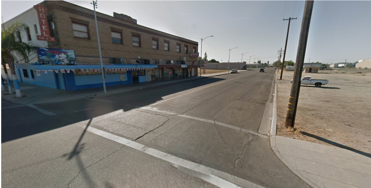
Figure 1. Photo in 2018 Before Construction of the ATP Project
