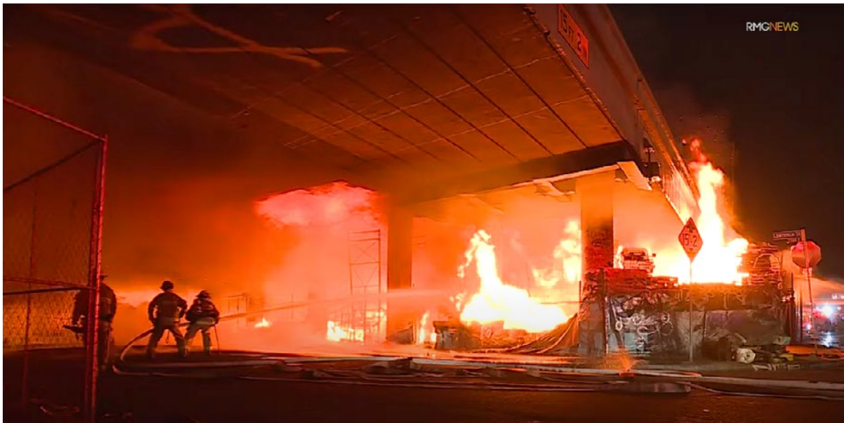
Figure 1. The image shows firefighters attempting to control the fire underneath the I-10 freeway structure.
