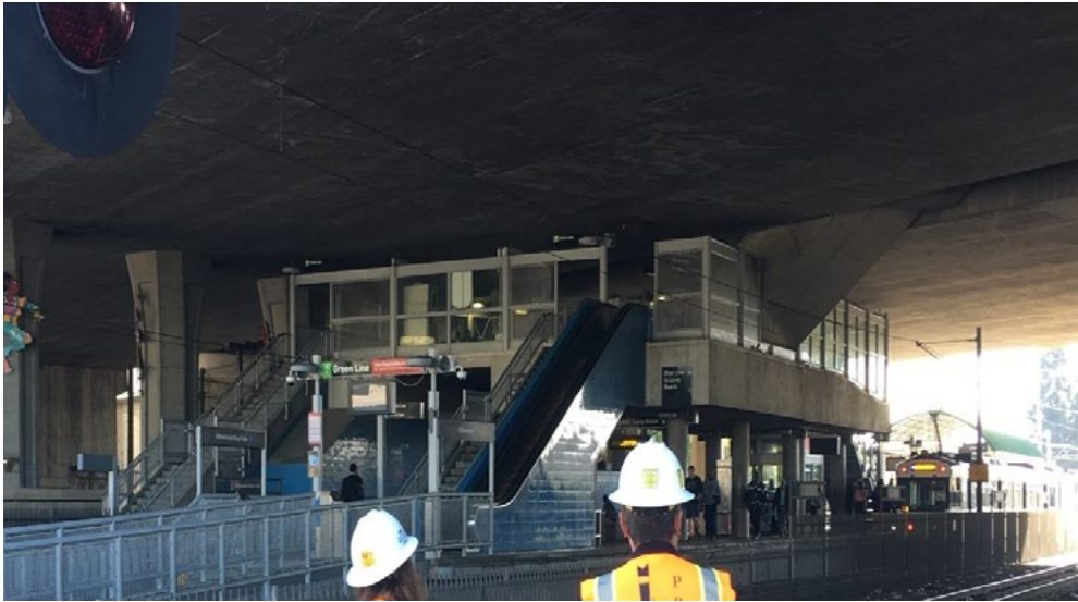
Figure 1. The image shows the mezzanine prior to construction.
