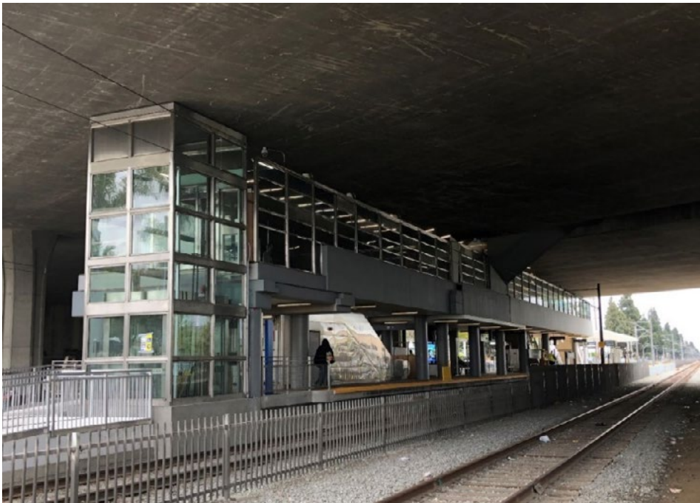
Figure 2. The image shows the extension of the mezzanine post construction.
